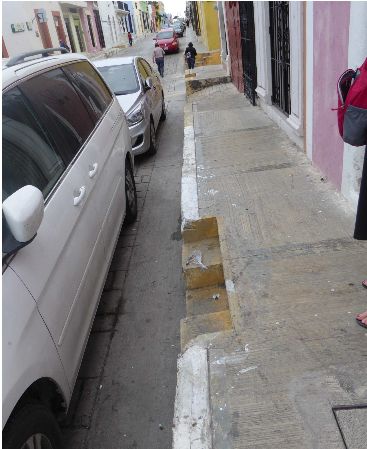
You've got to love Mexico. When the streets slope down for drainage, no point in sidewalks following. Just add steps! Note the lady in dark clothes at the end of the block where the curb is about 4 feet high and 5 steps.
